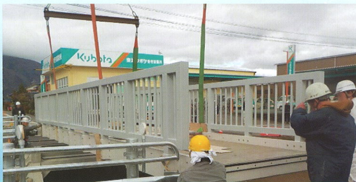
Installation in progress
