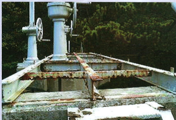
Existing operation bridge
