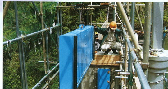
Installation in progress using only simple installation tools
