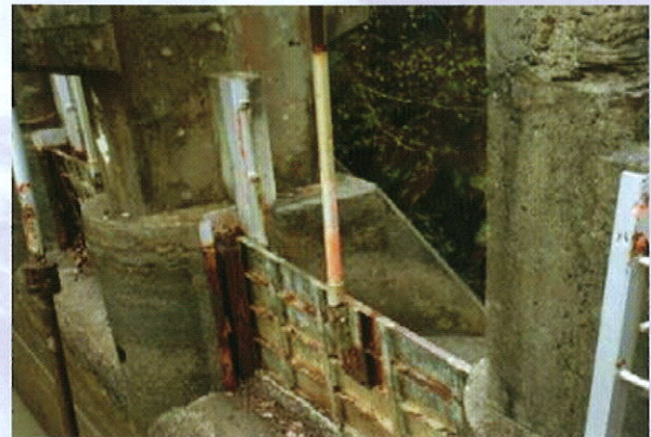
Existing steel gate leaf
