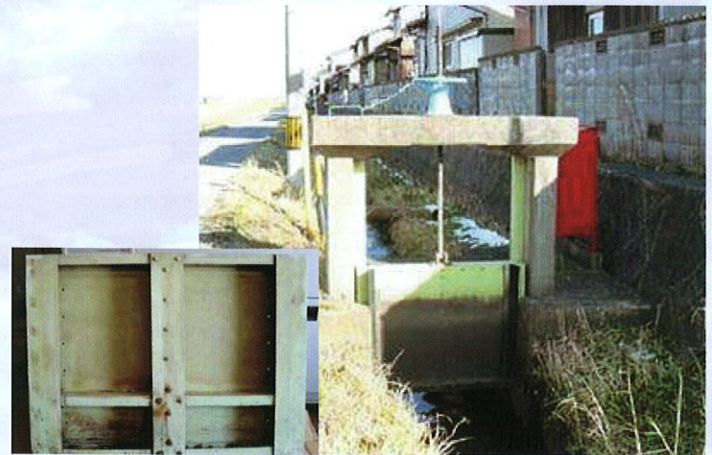
FRP hydraulic gate (enlarged view of gate leaf)
